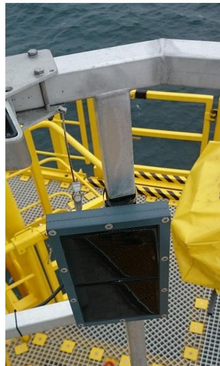
*Installed POE network antenna in an offshore wind park.*
